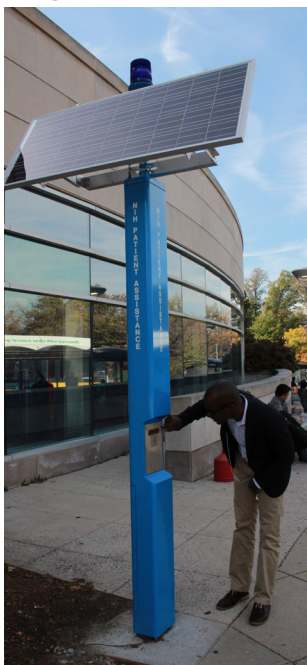
The use of a solar-powered device to run the phone eliminated the need for disruptive and costly construction.
