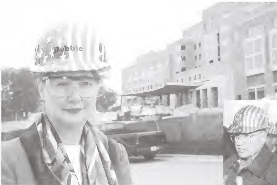
Hospital Activation Coordinator Debbie Byram often tours the CRC construction area. Her patriotic hardhat is similar to that worn by Vice President Dick Cheney (inset) in the aftermath of the September 11 tragedy. Inset photo from Dec. 31, 2001, Time magazine.
