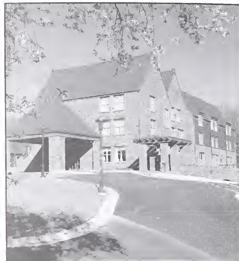
The exterior of the newly completed Edmond J. Safra Family Lodge.
