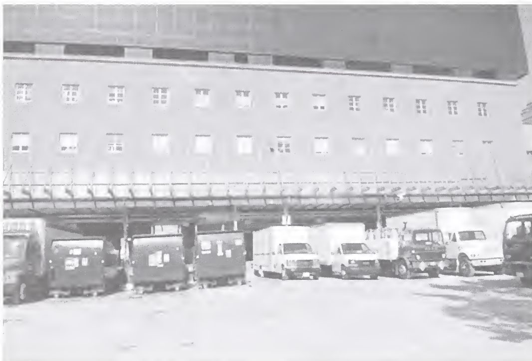
A 21-foot ramp connects the B2 loading dock to the CRC. The Loading Dock Management Services was implemented in anticipation of the opening of the CRC.
