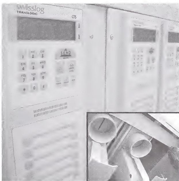
The new carrier panels are sophisticated, but the interface is remarkably easy to use. Inset: Tube retrieval slots can withhold carriers until a PIN is entered.
