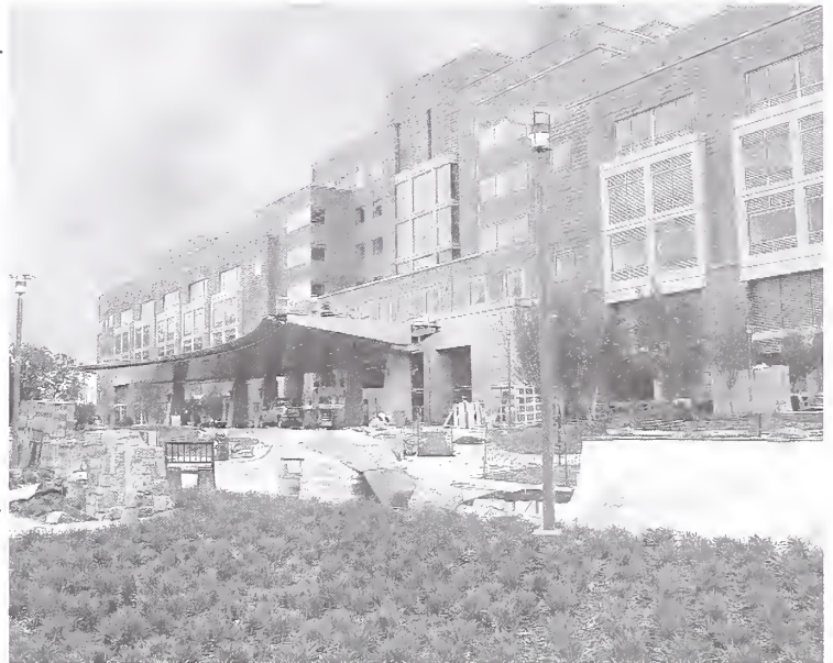
The CRC entrance and the landscaping are nearly complete.
