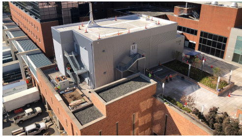
New Center for Cellular Engineering facility at the NIH Clinical Center.
